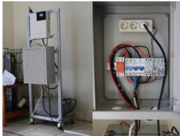
Figure 6. Control Panel Installation
